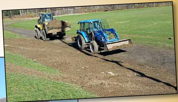
The Town of Great Valley front loader is helping the maintenance staff use excess dirt/gravel from the new softball field to backfill the bank overlooking the football field. The goal is to reduce the drop off in front of the Press Box/Concession Stand and create a more gradual slope for the safety of our spectators. We plan to fill part of the area now and finish it in the spring after there is time for the dirt to settle.
